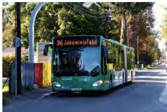
Ladestation für Elektrobusse der Grazer Verkehrs- betriebe, Andersengasse Charging station in Andersengasse for electric buses of the public transport authority of Graz
